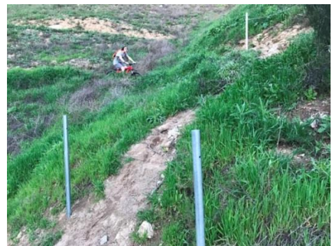
Trail damage caused by cutting a switchback Fences were installed for restoration.
